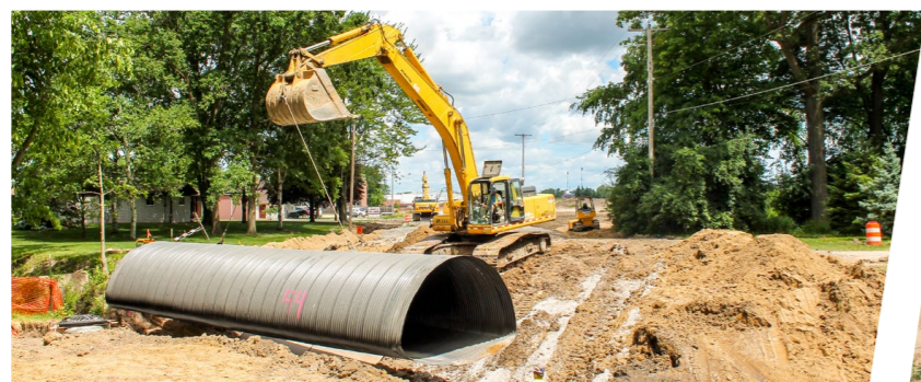
8 Stronger, Safer Roads: Kochville Township's Davis Road Receives Upgrades
