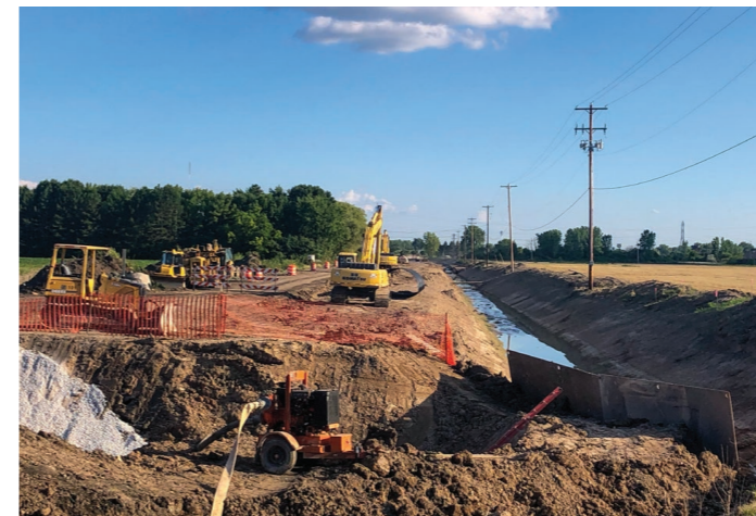
/ Davis Road during construction.
