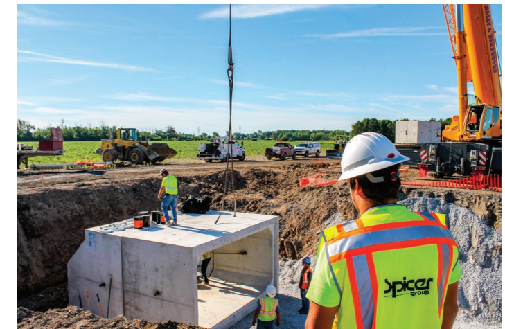
/ New box culverts being installed along Davis Road.
