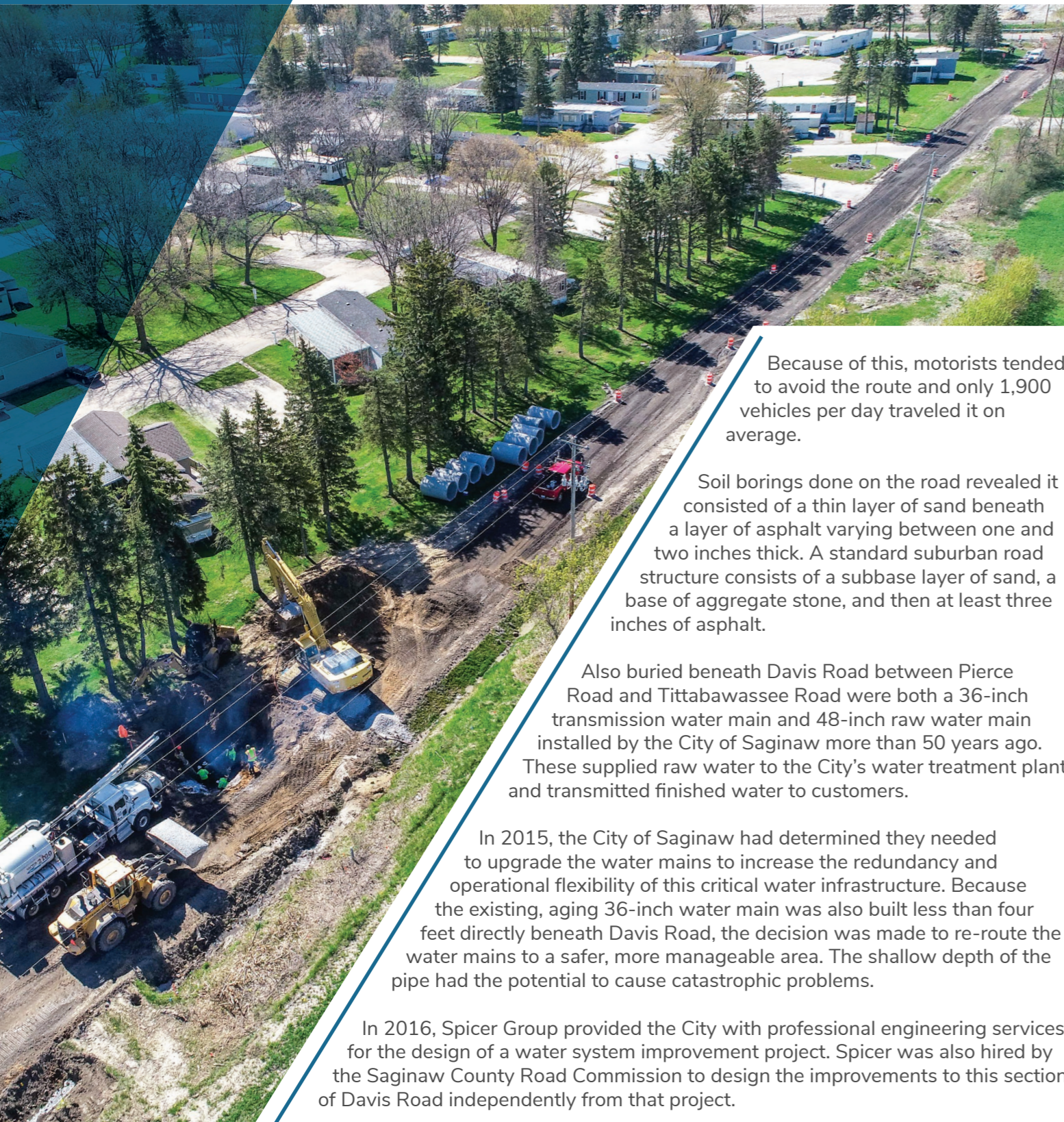
/ Aerial view of Davis Road under construction.
