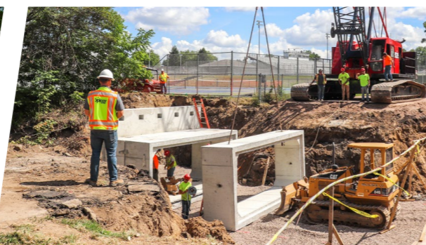
12 Improvements Along the John Earl Drain Reduce Flooding in Eaton County
