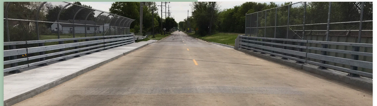
New Concrete Deck, Approaches and Guardrail
