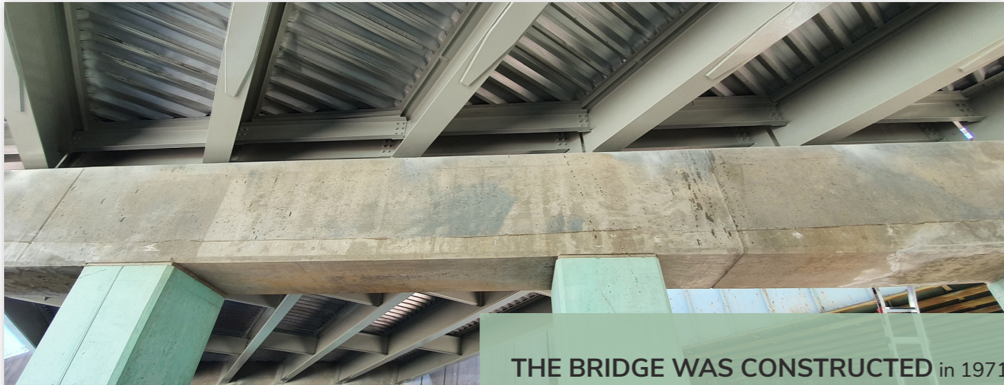
Newly Painted Beams and Steel Corrugated Decking
