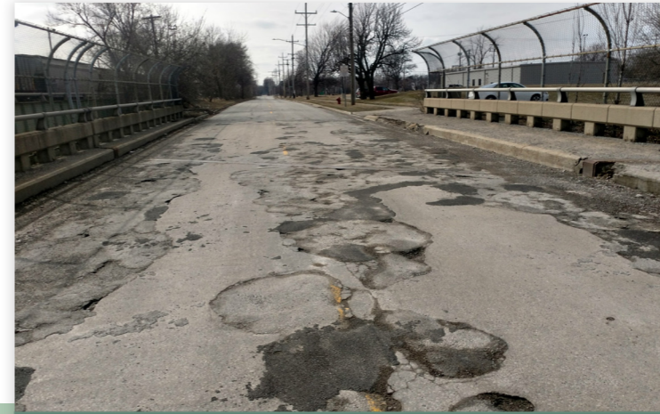
Norman St. Bridge Deck Before the Replacement
