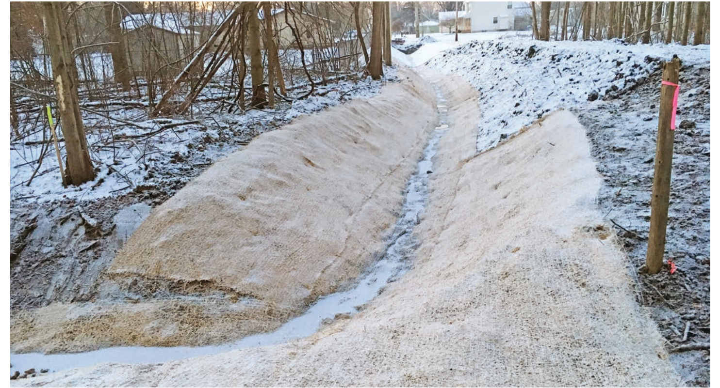
New open-drain portion of the project.
