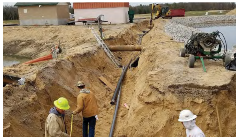
Blower pipe installation around lagoon cell
