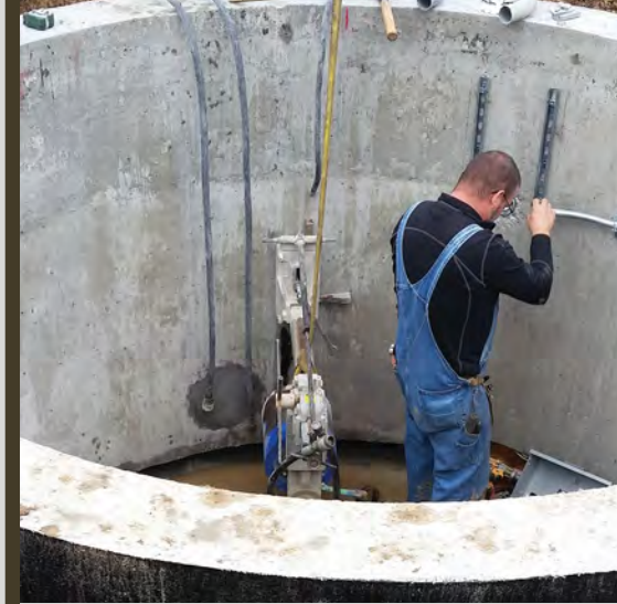
Above and below: PRV vault installation
