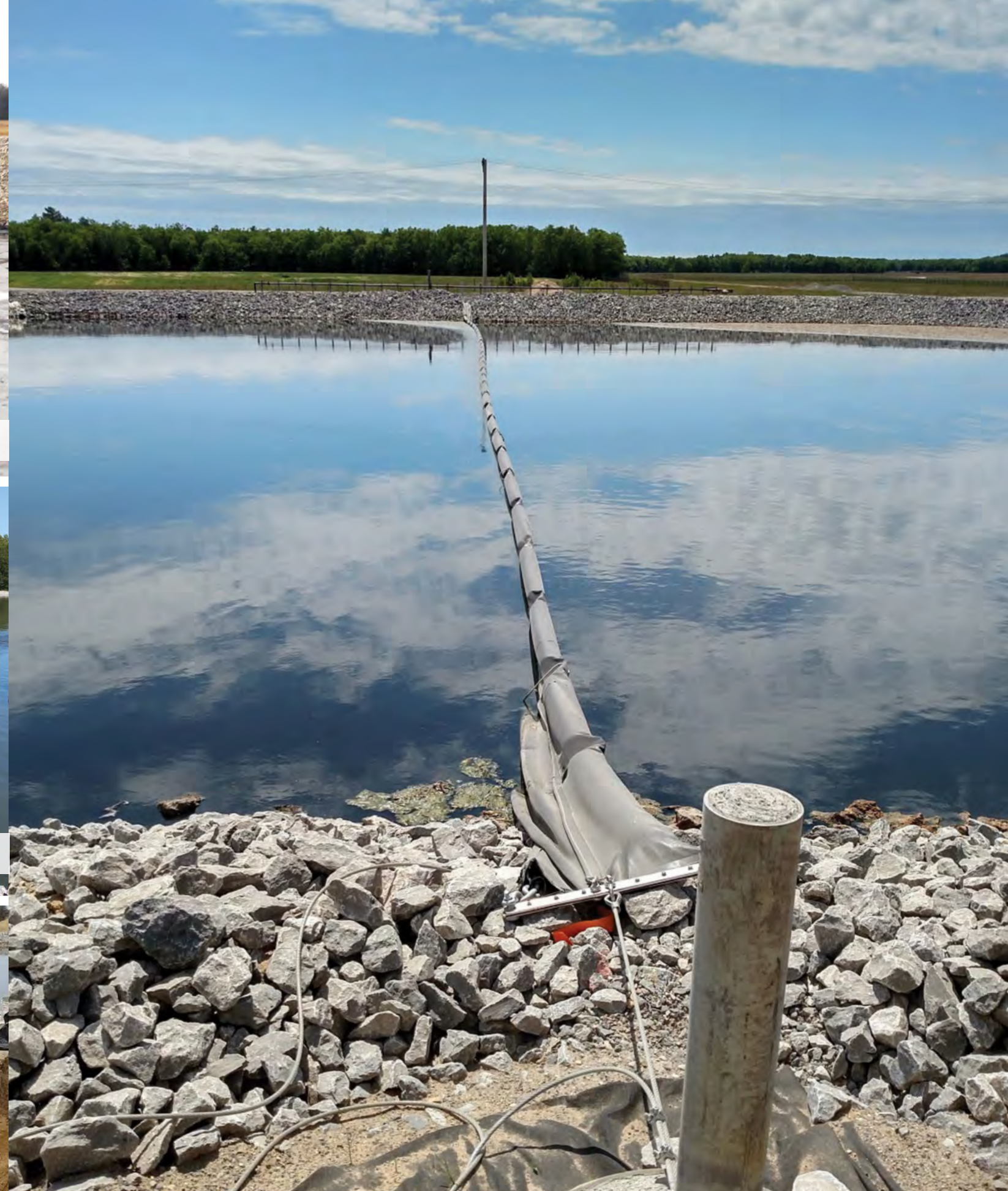
Finished lagoon cell with baffle curtain
