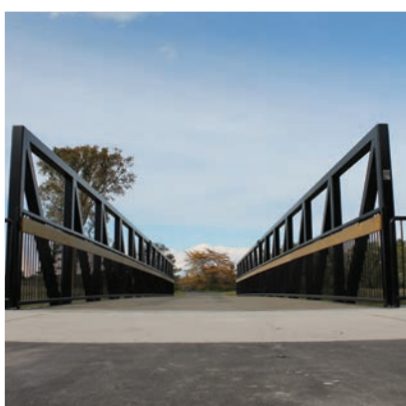
Sunrise Side Path Extension, Alabaster Township, $718,160 MDOT TAP Grant
