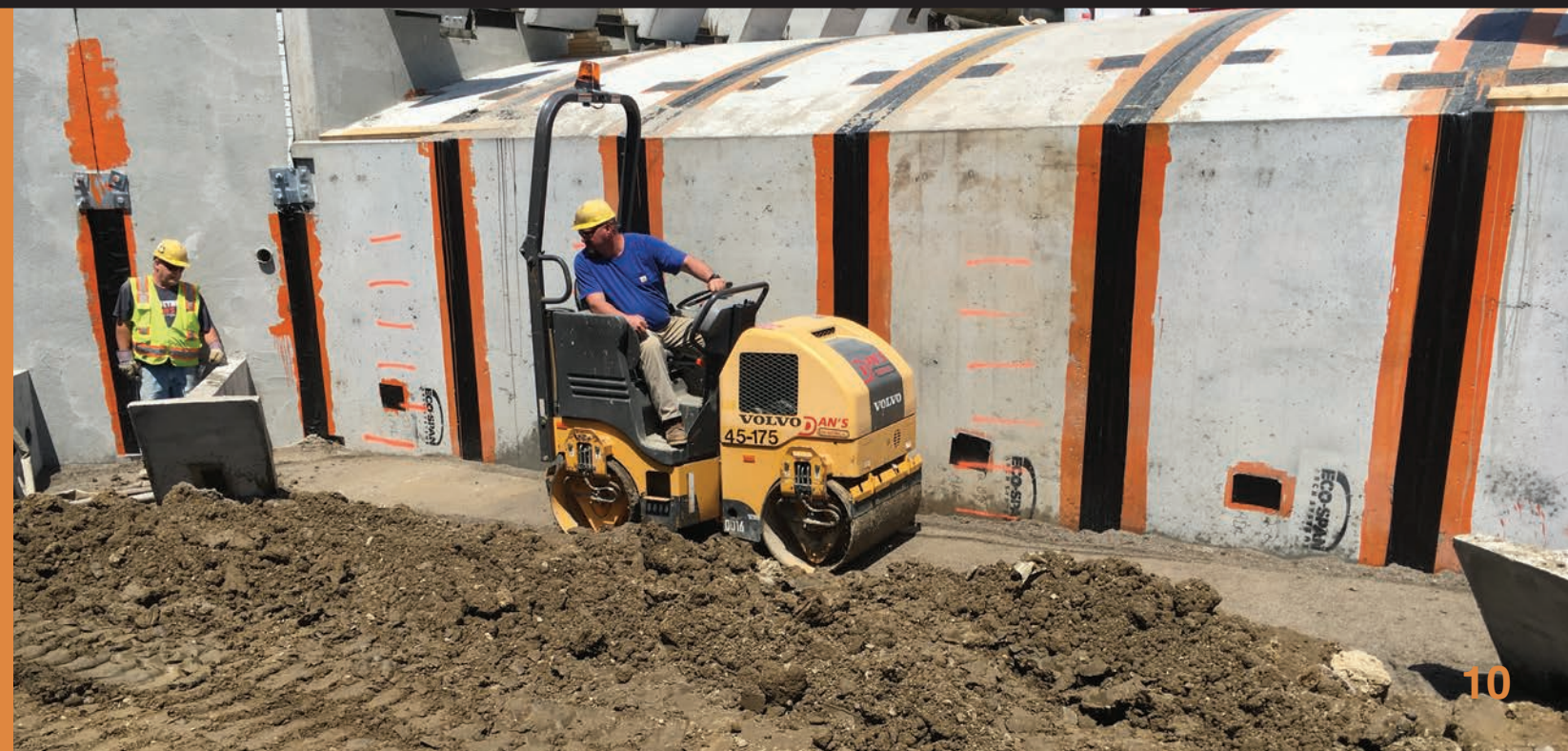
COMPACTING SAND FILL AROUND THE ARCH BRIDGE IN TYLER POND
