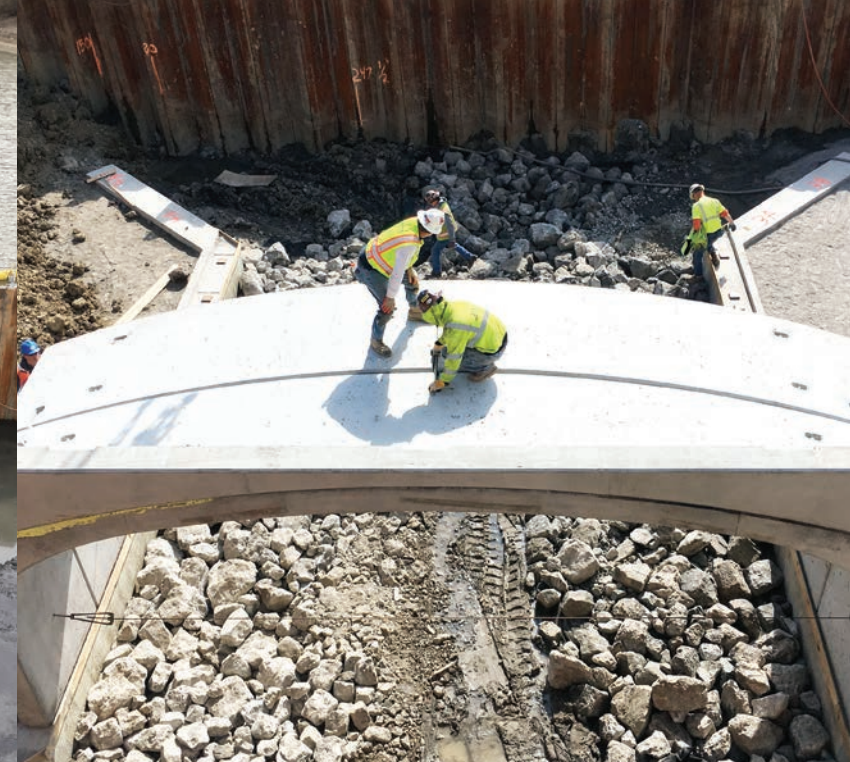
SETTING A PRE-CAST ARCH BRIDGE
