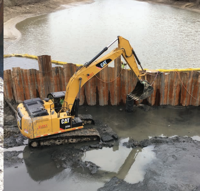
INSTALLING OF SHEET PILING AT COFFER DAM
