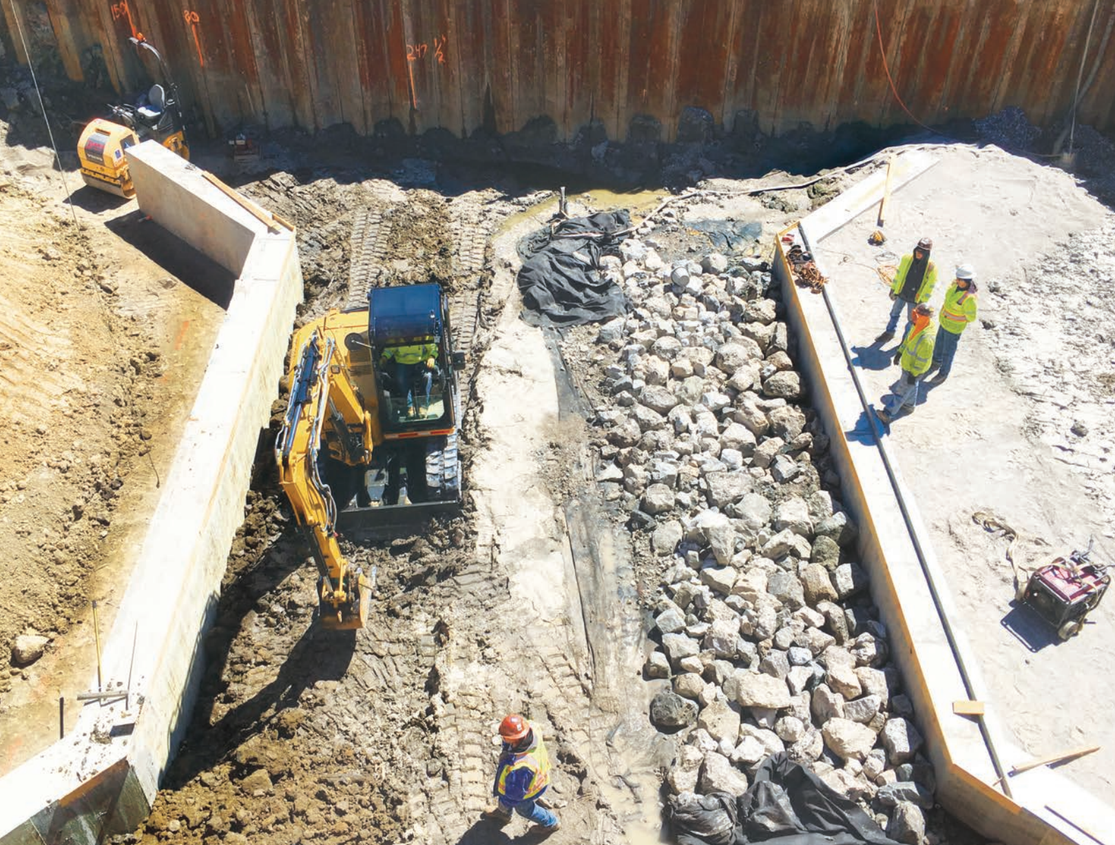
INSTALLATION OF RIP RAP TO PROTECT THE NEW CULVERT'S ARCH BRIDGES
