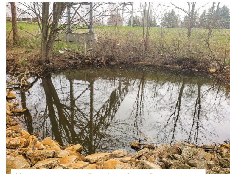
Upstream water pooling along the project waterway.
