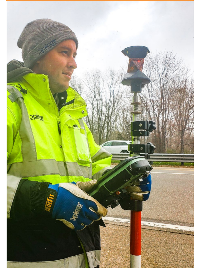
Spicer Group's Survey Crew Chief Jared Johnson begins mapping the edge of US-31.
