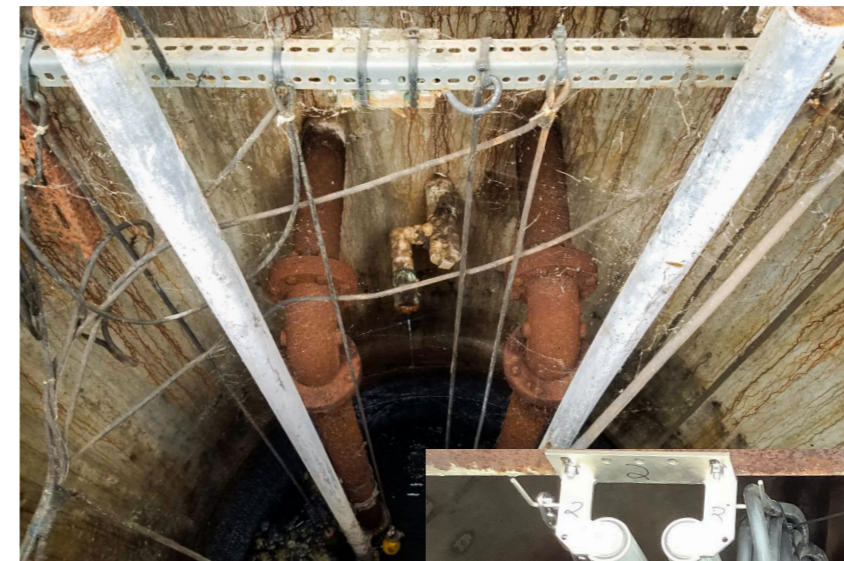
Former pump station wet well.
