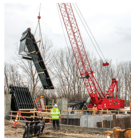
New Duperon® self-cleaning trash rack being installed.
