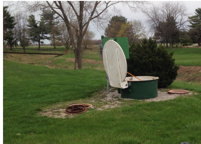
Original pump station structure in the Village of Akron.
