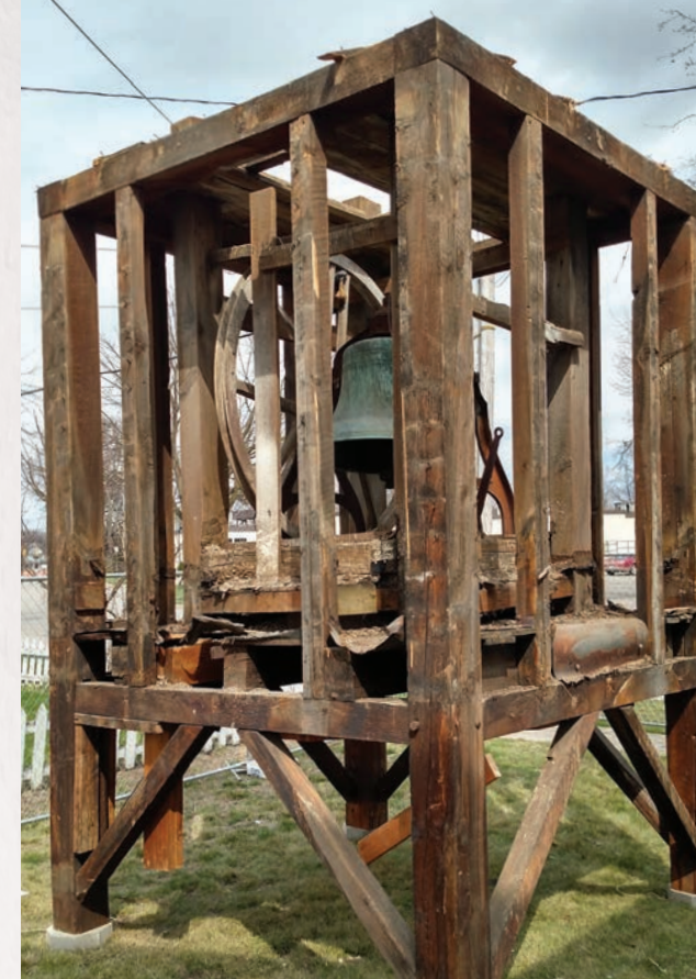
The 130-year-old bell tower that was removed from the Creative Passions building now sits on display on the front lawn.
