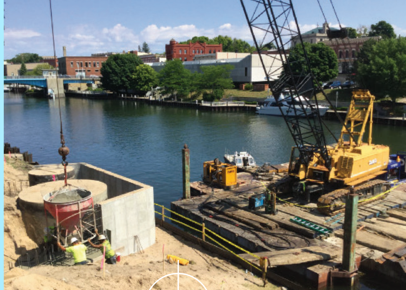
Above: Pouring concrete from a barge.
