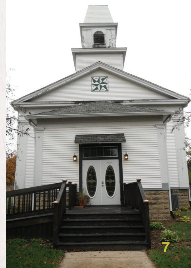
The 150-year-old Creative Passions building prior to the removal of its bell tower.
