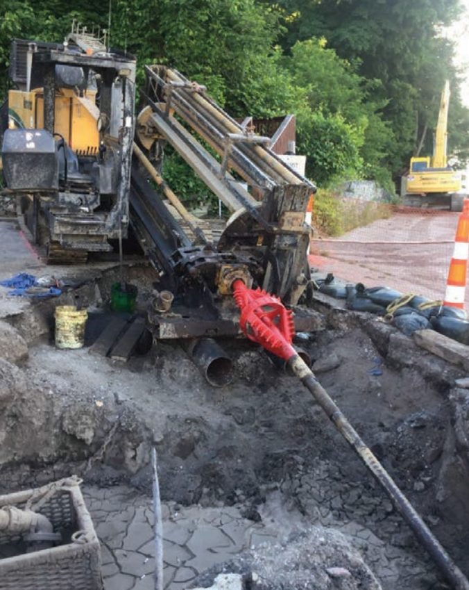
Above: Drilling beneath the Manistee River.
