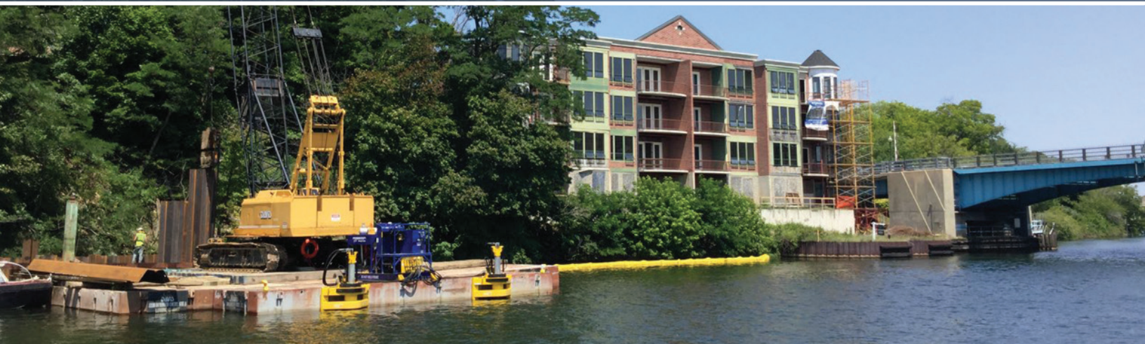
Below: Installing the new sheet pile wall from a barge.
